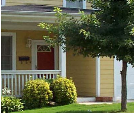
Steps at all entrances
