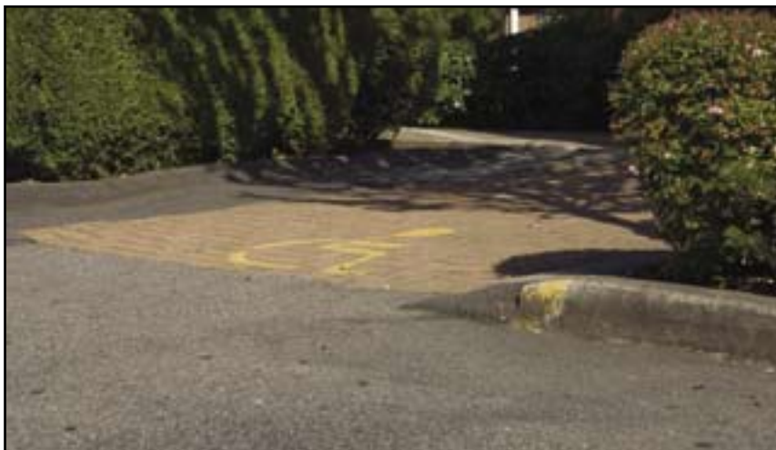
Parking Lot with Wheelchair Accessibility - Maple Ridge, B.C. photo credit: Natasha MacArthur
