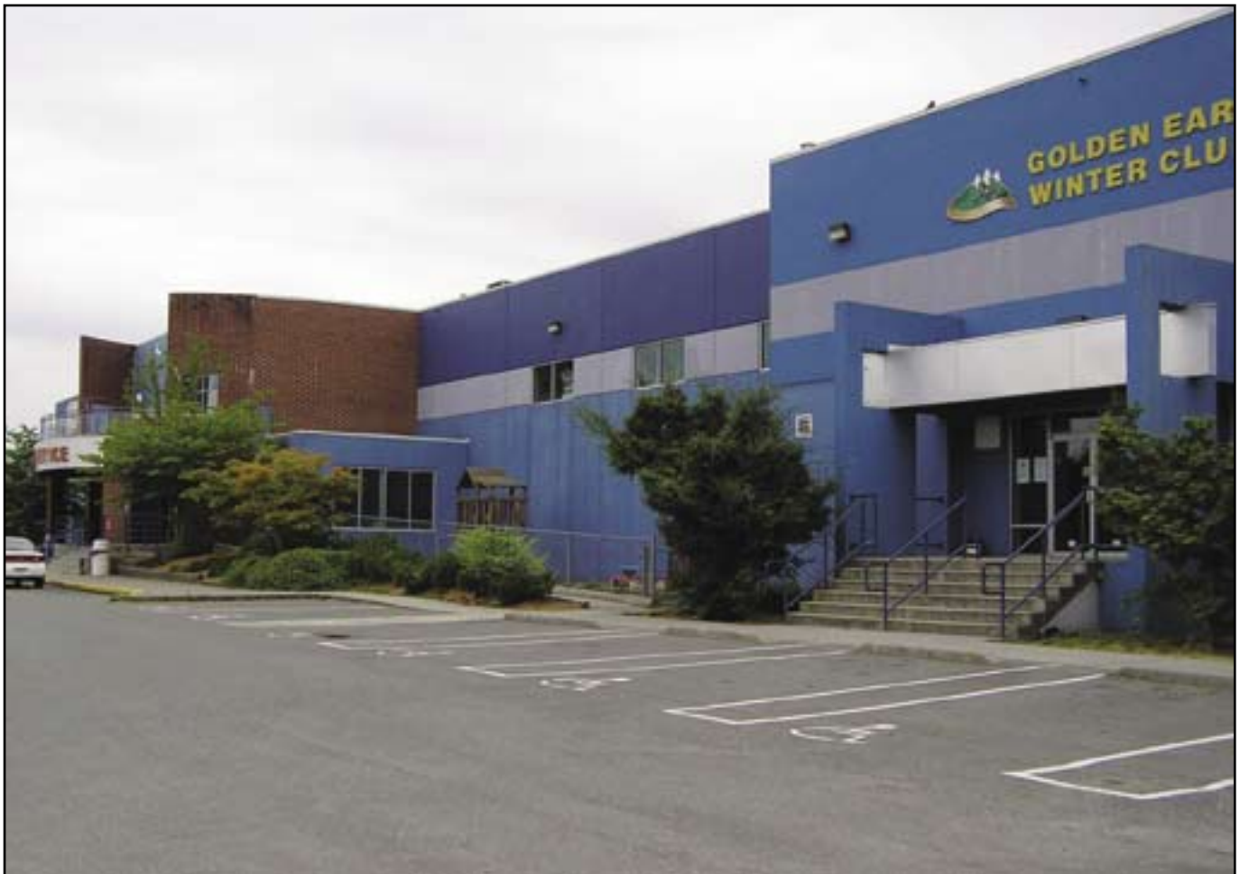
Accessible Parking, Building Entries and Drop-Off/Pick-Up Areas Planet Ice and Golden Ears Winter Club, Maple Ridge, B.C. / photo credit: Donna Rodman
