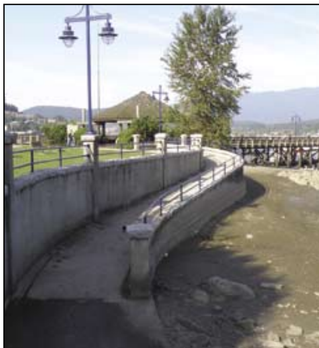
Beach Access Ramp – Rocky Point, Port Moody, B.C. photo credit: Petra Frederick
