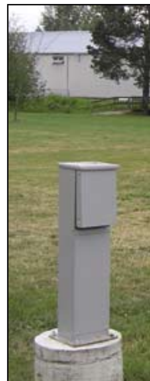
Battery Recharge Outlet – Maple Ridge Fairgrounds, Maple Ridge, B.C. photo credit: Donna Rodman
